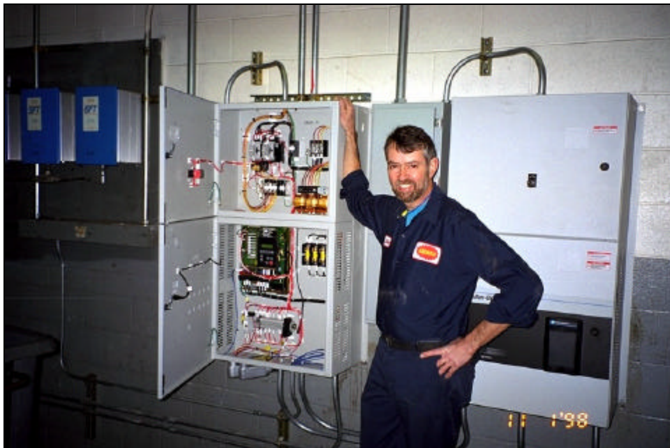
Figure 2: Darigold Dairy Milk Cooler VFDs
